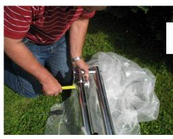
Setting of the overhanging of the pool edge on the spacer
